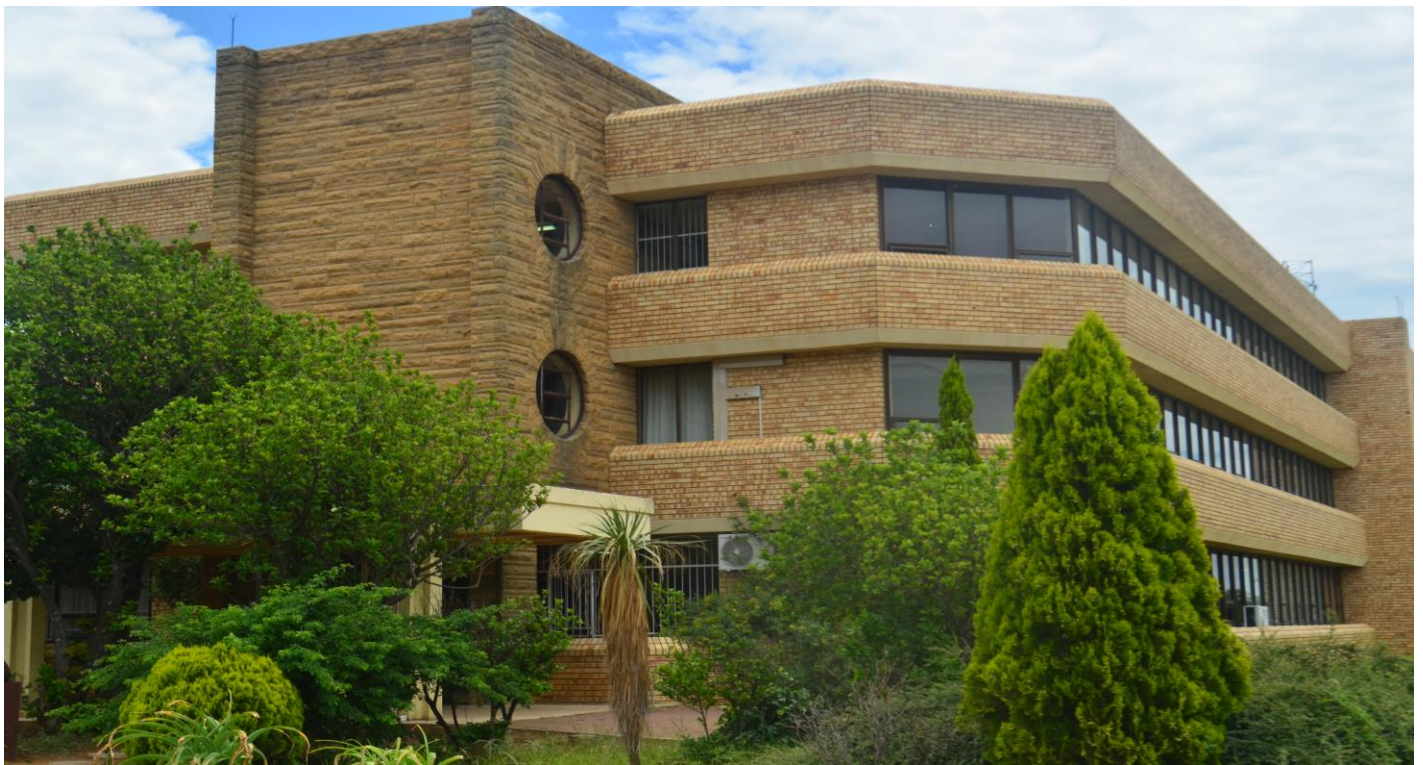
THABO MOFUTSANANYANA DISTRICT MUNICIPALITY OFFICES. OLD PARLIAMENT BUILDING.
